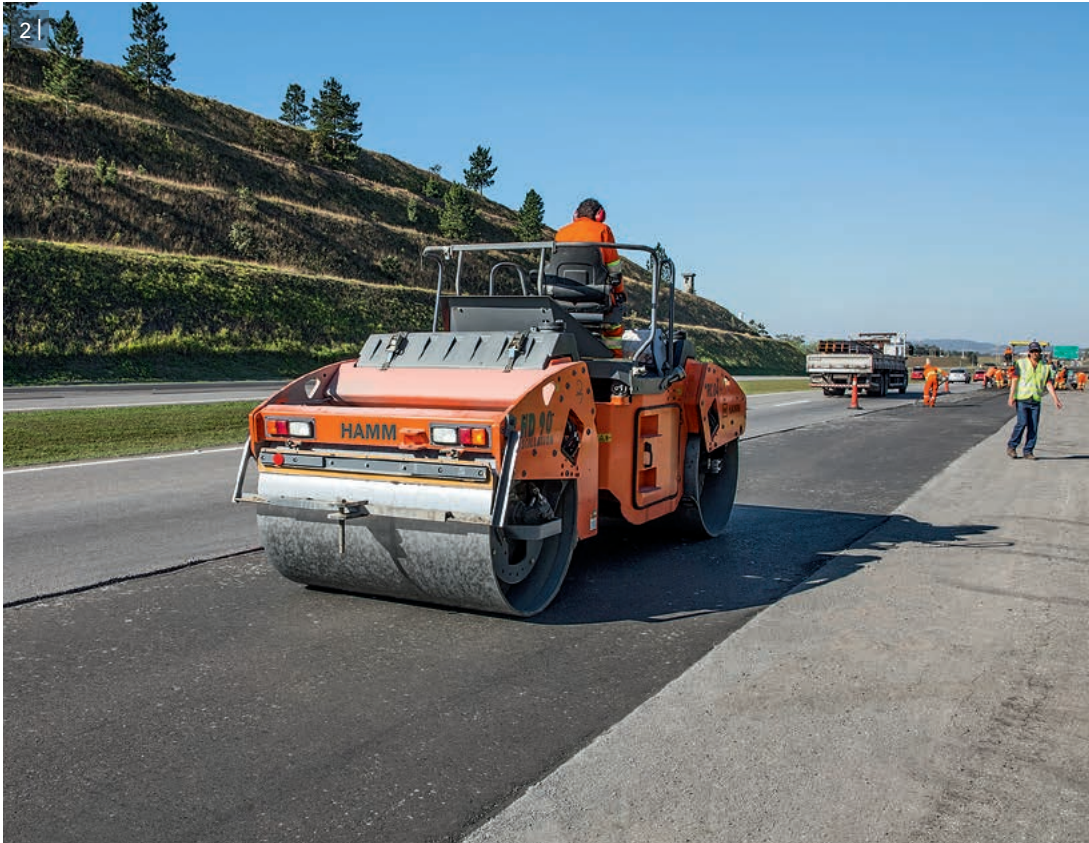
3 | Two-lane carriageway without surfacing, produced from cold mix.
