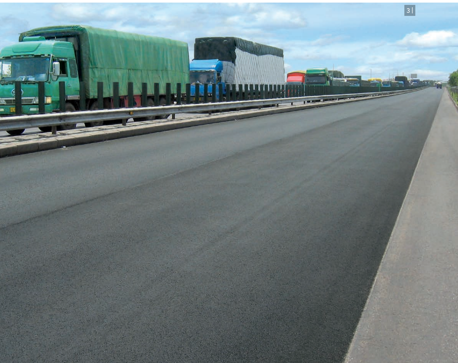
3 | Two-lane carriageway without surfacing, produced from cold mix.
