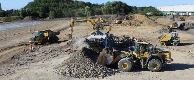
All asbestos materials were doublebagged for off-site disposal. The processed soils were then validated by means of laboratory testing and backfilled below the site access road and car parks. The operation was carried out under the Control of Asbestos Regulations 2012 with an asbestos analyst carrying out air monitoring.
